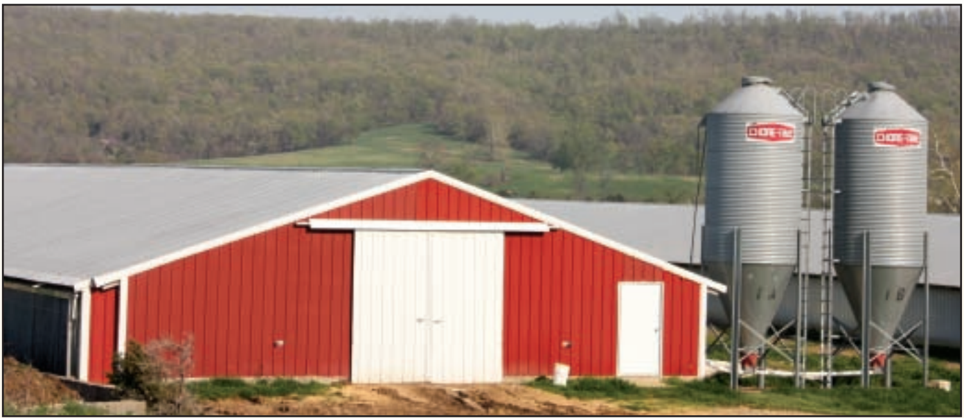
Four of Jerry Hutton's poultry houses are being used in a University of Arkansas pilot energy efficiency project funded by an ARRA stimulus grant.
